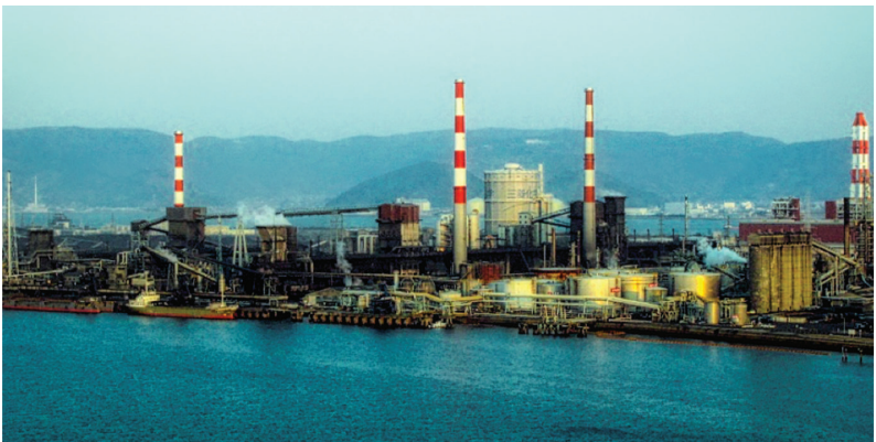
Petrochemical complex located at Okayama
